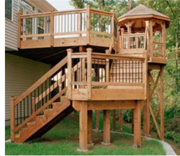
Learn deck inspection musts.
